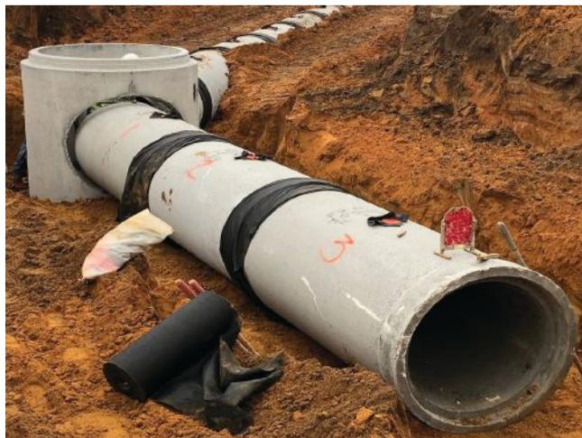
Foley Products shipped 12- to 48-in. diameter concrete pipe, plus precast inlets, junction boxes, catch basins and headwalls for storm sewer infrastructure on a private Alabama industrial site.
